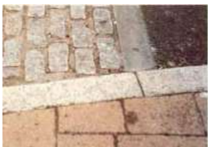
Victorian paving bricks, conservation kerbing, grey or brindle “drivesett” blocks, stone setts, cobbles and tarmac are preferred materials than that of modern day block-paving
